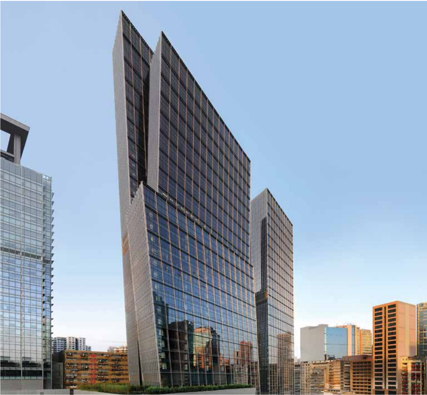
Landmark East Building, Hong Kong
